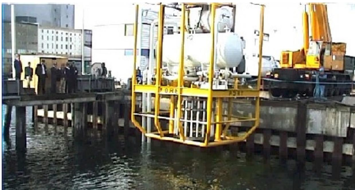
**Figure 3 – Demonstrating the ease of installation and commissioning of Alpha Thames' prototype System-Module during its in-water trials**
